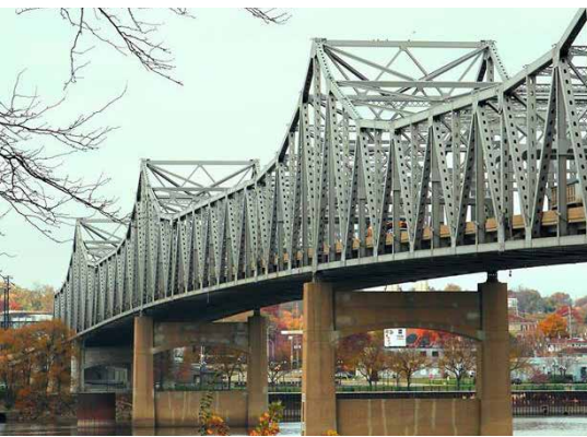
A new volunteer initiative to re-light the Murray Baker Bridge has been announced. To learn more visit: lightitup74.wixsite.com/fliptheswitch .
